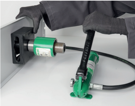
Making the cut-out with a punch.
